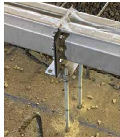
We are particular about ensuring easy installation and quick adjustment, where our anchorage points are a strength. They make the channel extremely stable with brackets every metre of the way. The top cover foil must remain in place during the entire process of casting and surfacing work to prevent concrete and other debris from entering in the slot.
